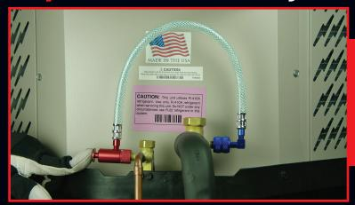
No manifold gauge or hoses needed Just Connect HI & LO -PUSH TO GO!
